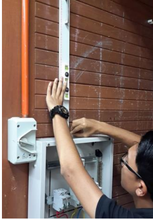
Figure 12: Student use EME as a ruler and create a line and an angle measurement using the built-in water level
